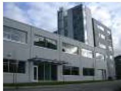
Clean Energy Research Centre
