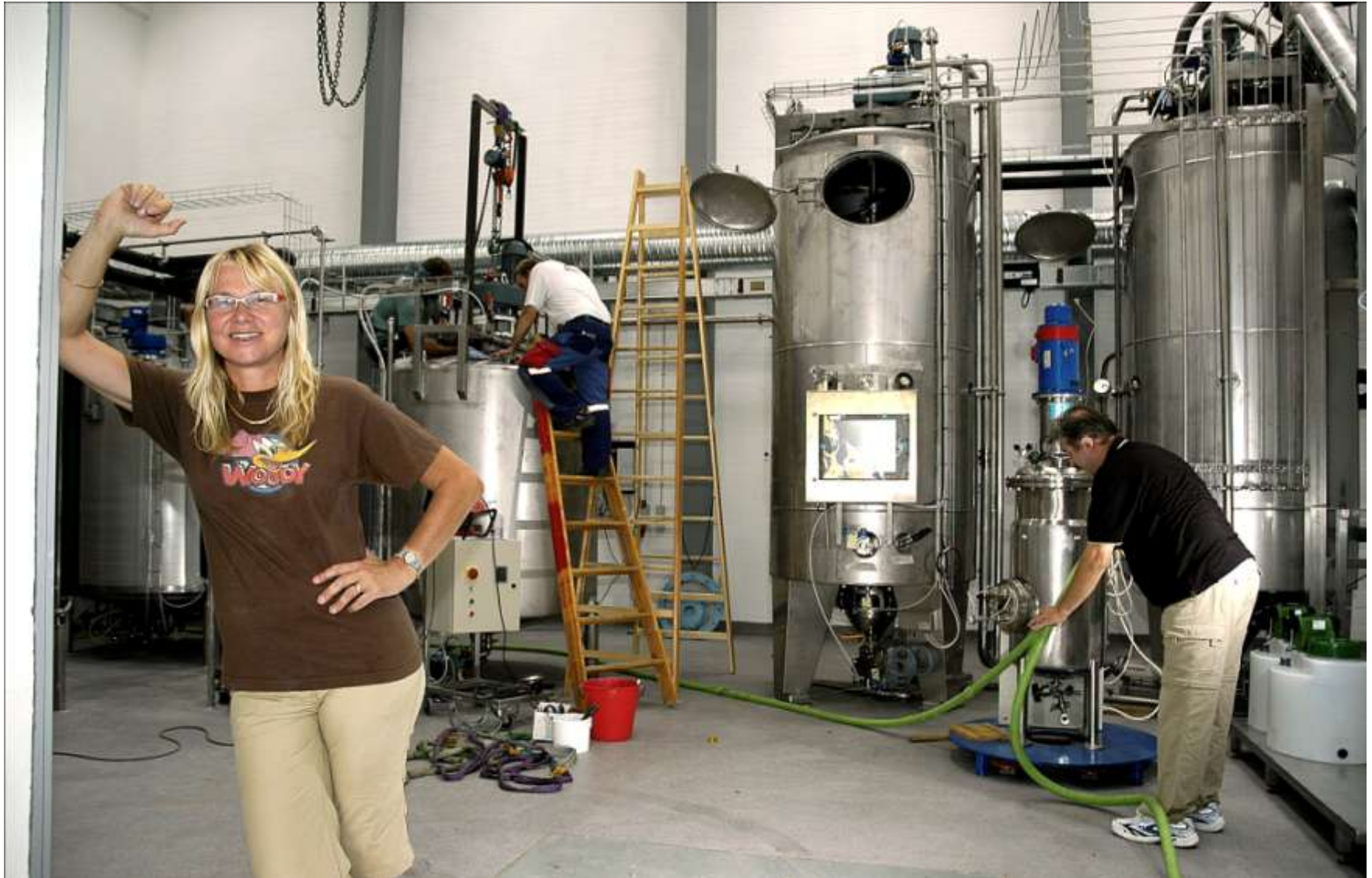
Pilot plant under construction
