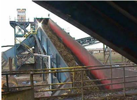
Figure B3. Moving material by a belt conveyor (Atchison and Hettenhaus 2003).
