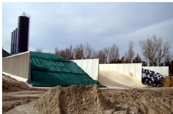
Figure A4. Covered material in concrete bunkers (source: http://www.hansonsilo.com/precast.php )
