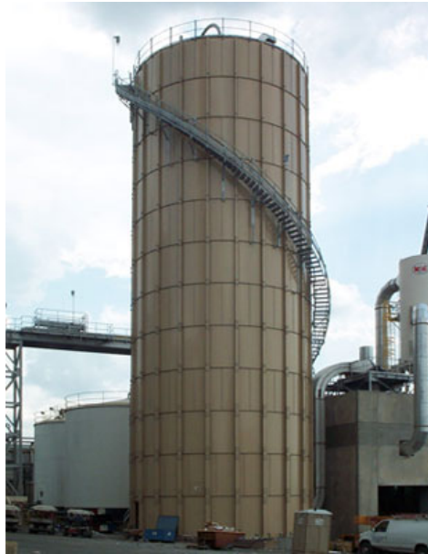
Figure A6. Silo for wood chips (source: http://www.columbiantectank.com/app_cat_sub_show.asp?id=23 ).
