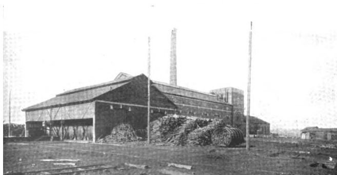
Figure 40. Older 200 t/day pyrolysis plant (12 retorts, each distilling 15 t/day) (Bunbury 1923).
